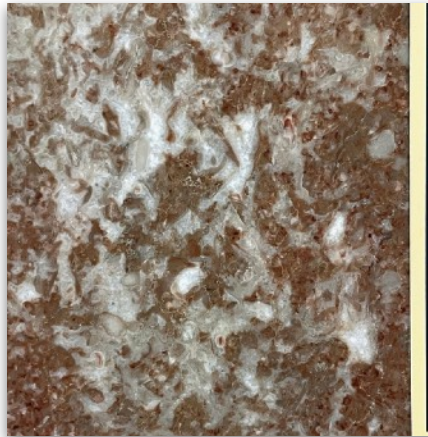
Figure 2. Close-up of Holston “marble” in the rotunda walls of Brehm Hall on the UT Martin campus showing “ramose (branching) colonies of bryozoans (white masses) within a strawberry-colored matrix (scale in cm, MAG photo, 2022).
